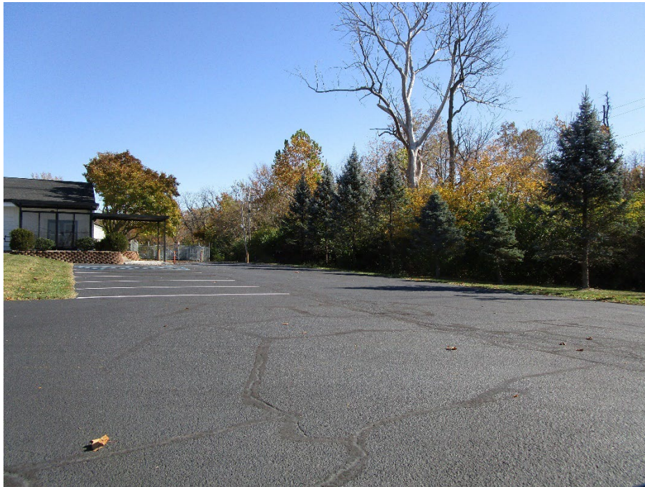
View of site looking southeast
