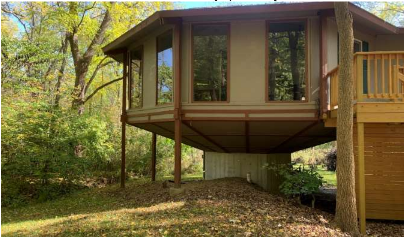
Photo of the northern building façade looking south.
