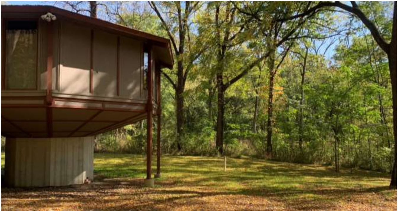
Photo of the proposed additional parking area on the south side.
