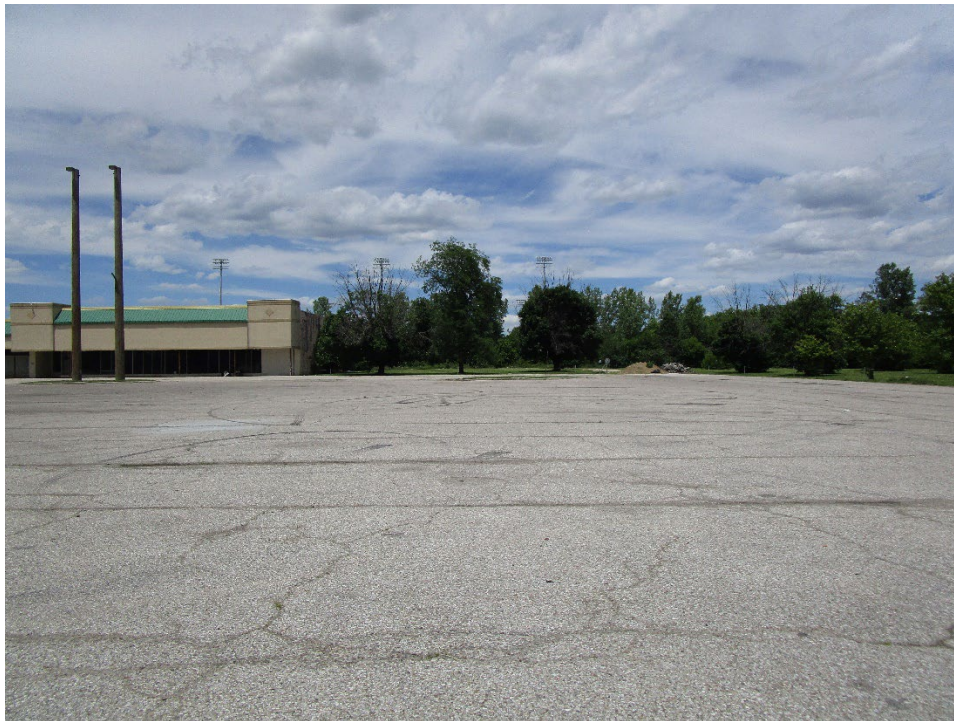
View of site looking north
