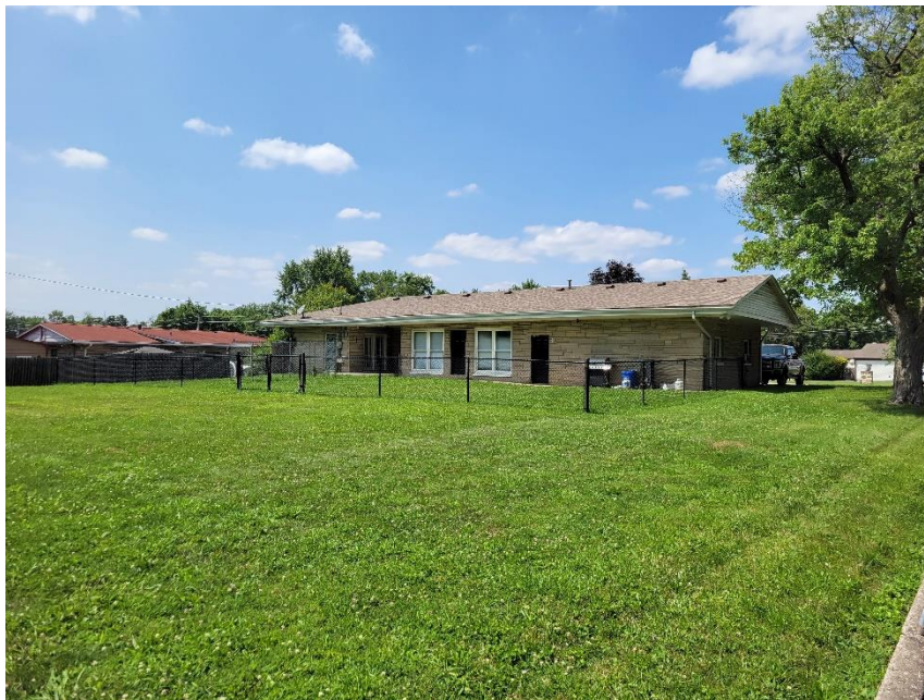
Photo 2: Primary Residence Viewed from Southeast
