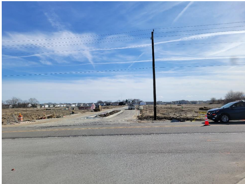
Photo 2: Previously Platted Section Viewed from North
