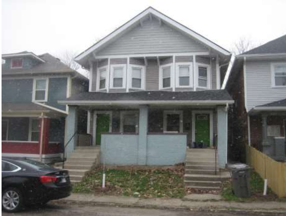
Subject site, proposed Lot 1 and 2, looking west.
