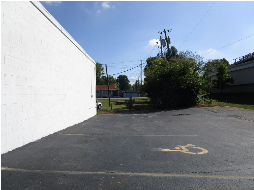
View of site looking east along southern boundary
