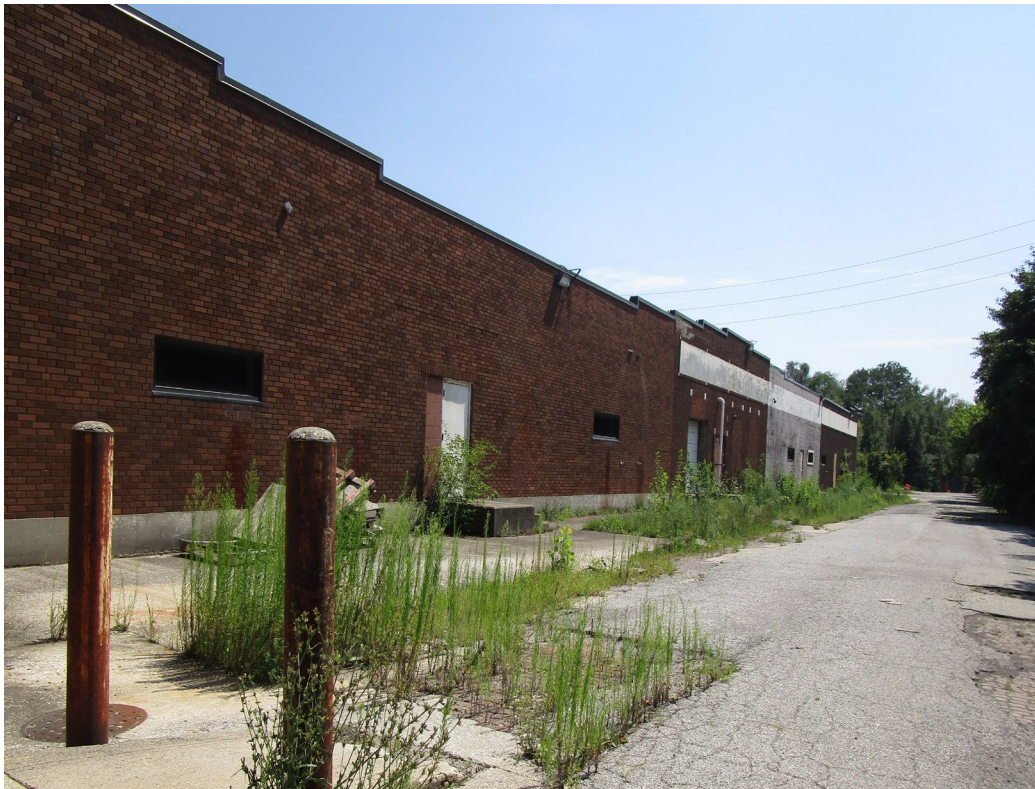
View of site looking southeast across Lewis Street
