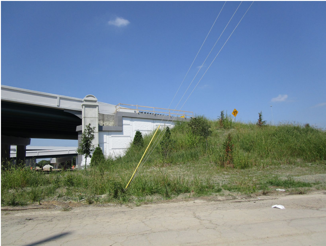
View from site looking north across East 13 th Street / I-70
