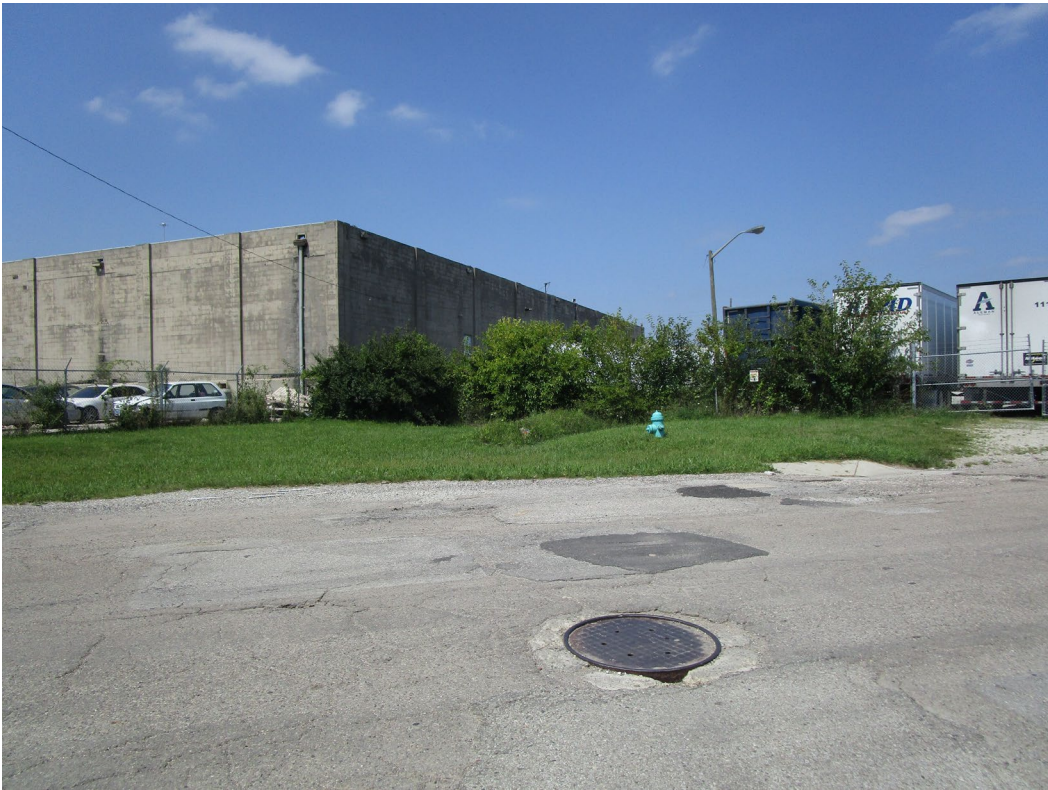
View of site looking northwest across Roosevelt Avenue
