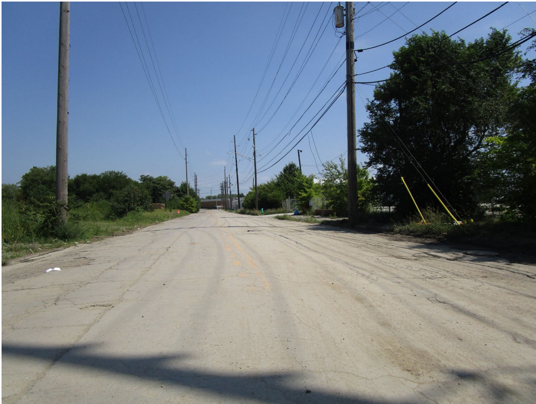
View looking east along East 13 th Street
