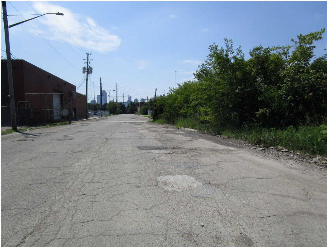
View looking west along Roosevelt Avenue
