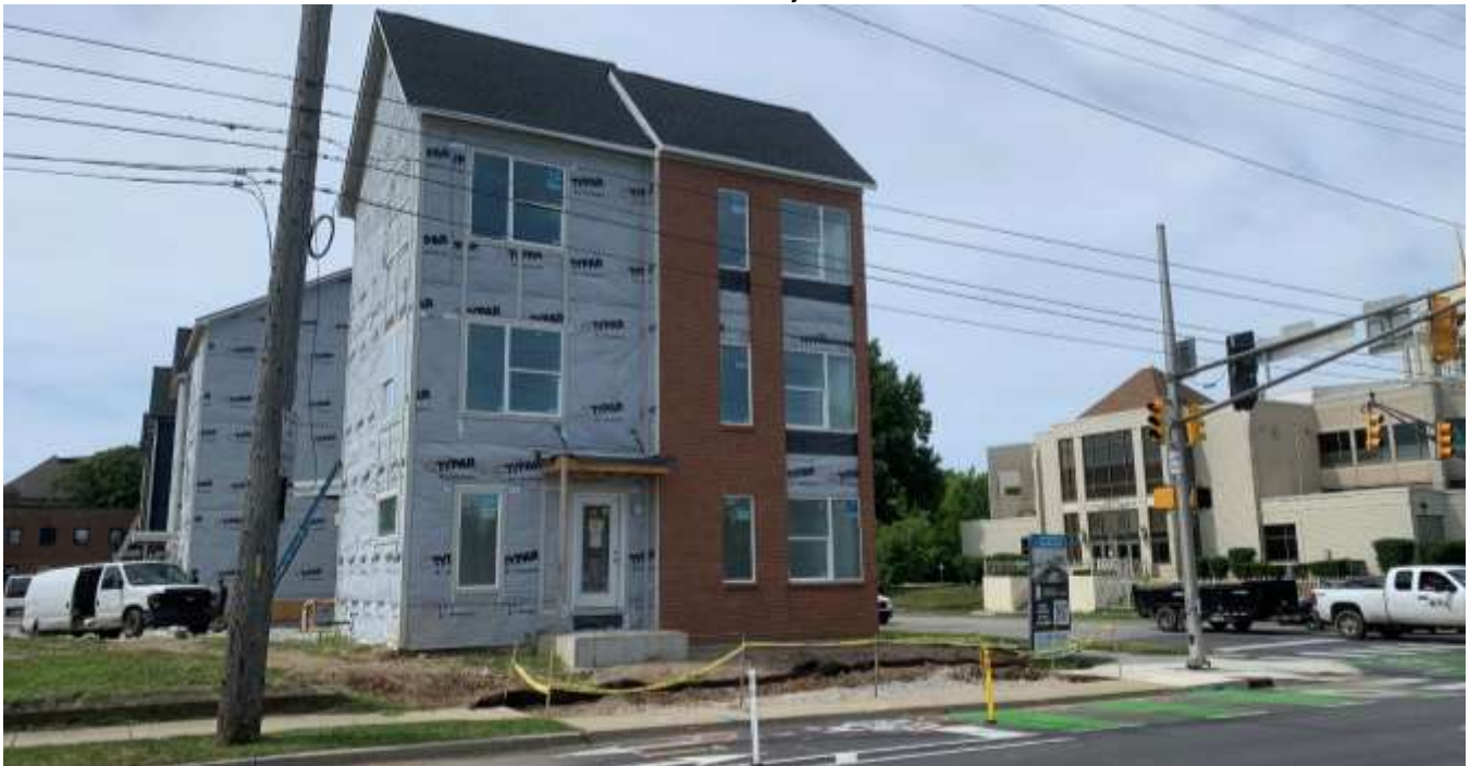
Photo of townhomes west of the site.
