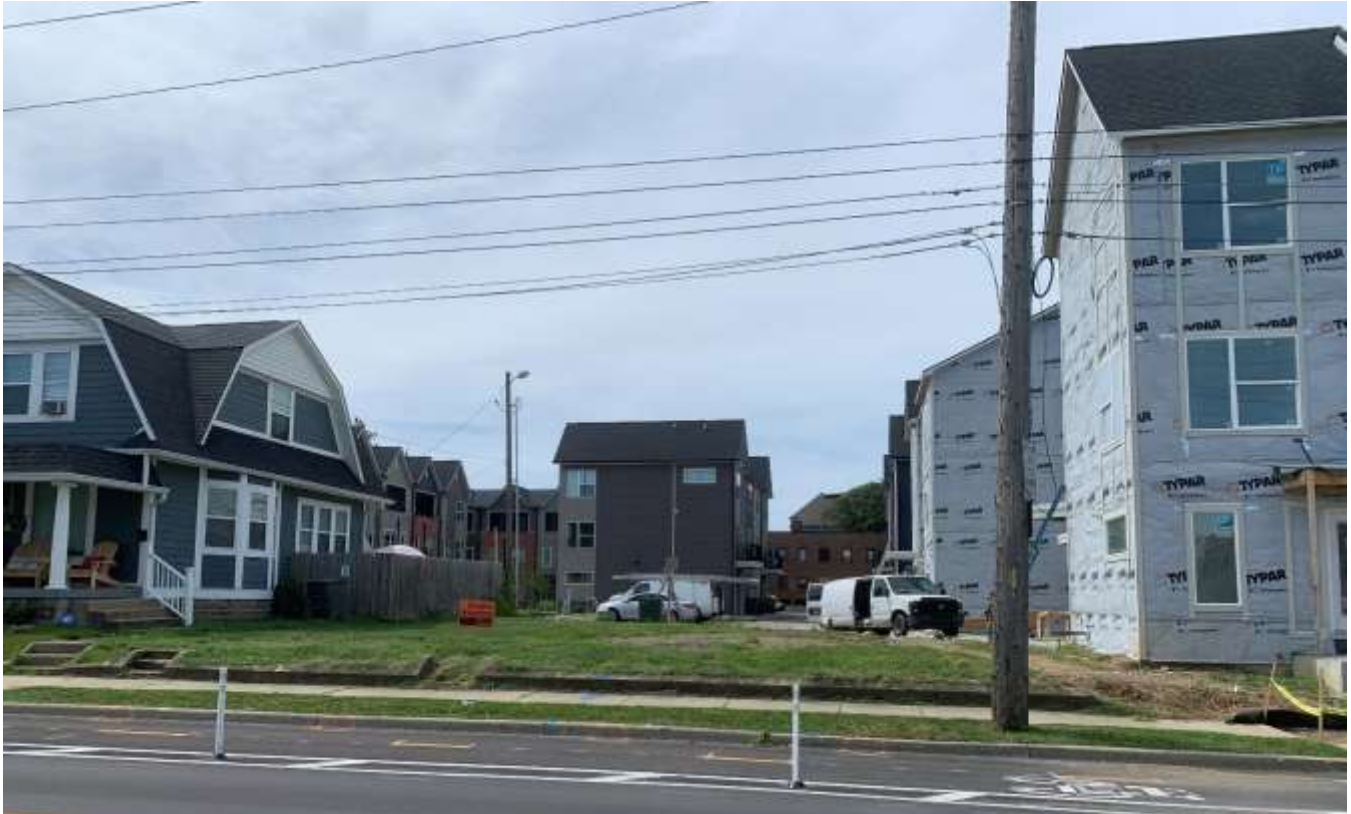
Photo of the subject site.
