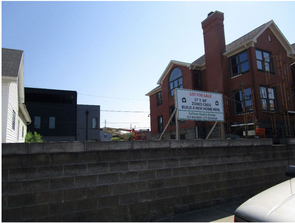
View of site looking east
