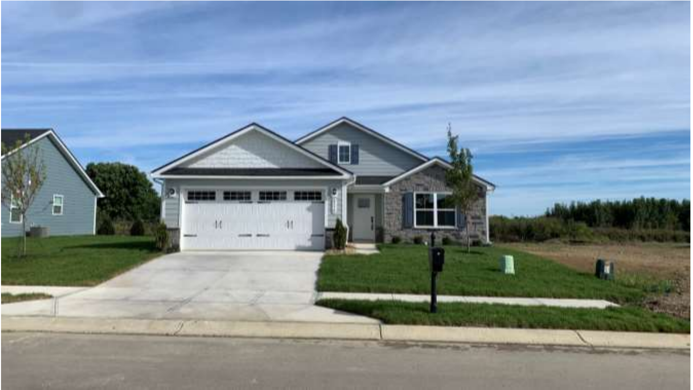
Subject site at 8550 Broad Street.
