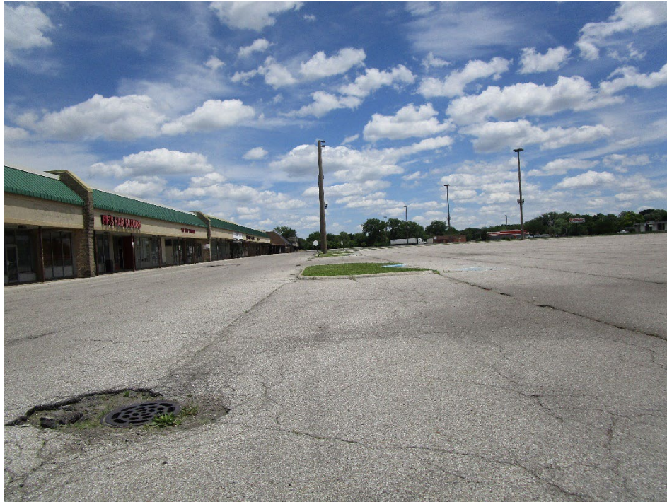
View of site looking east along existing structure
