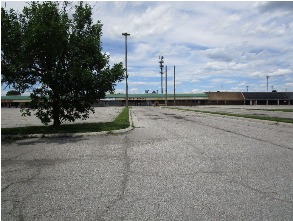
View of site looking north
