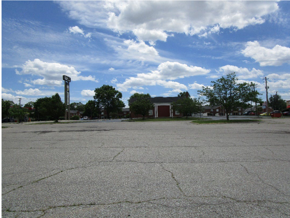
View from site looking south
