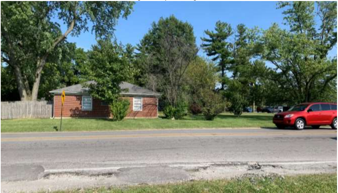
Photo of the single-family dwelling east of the site.
