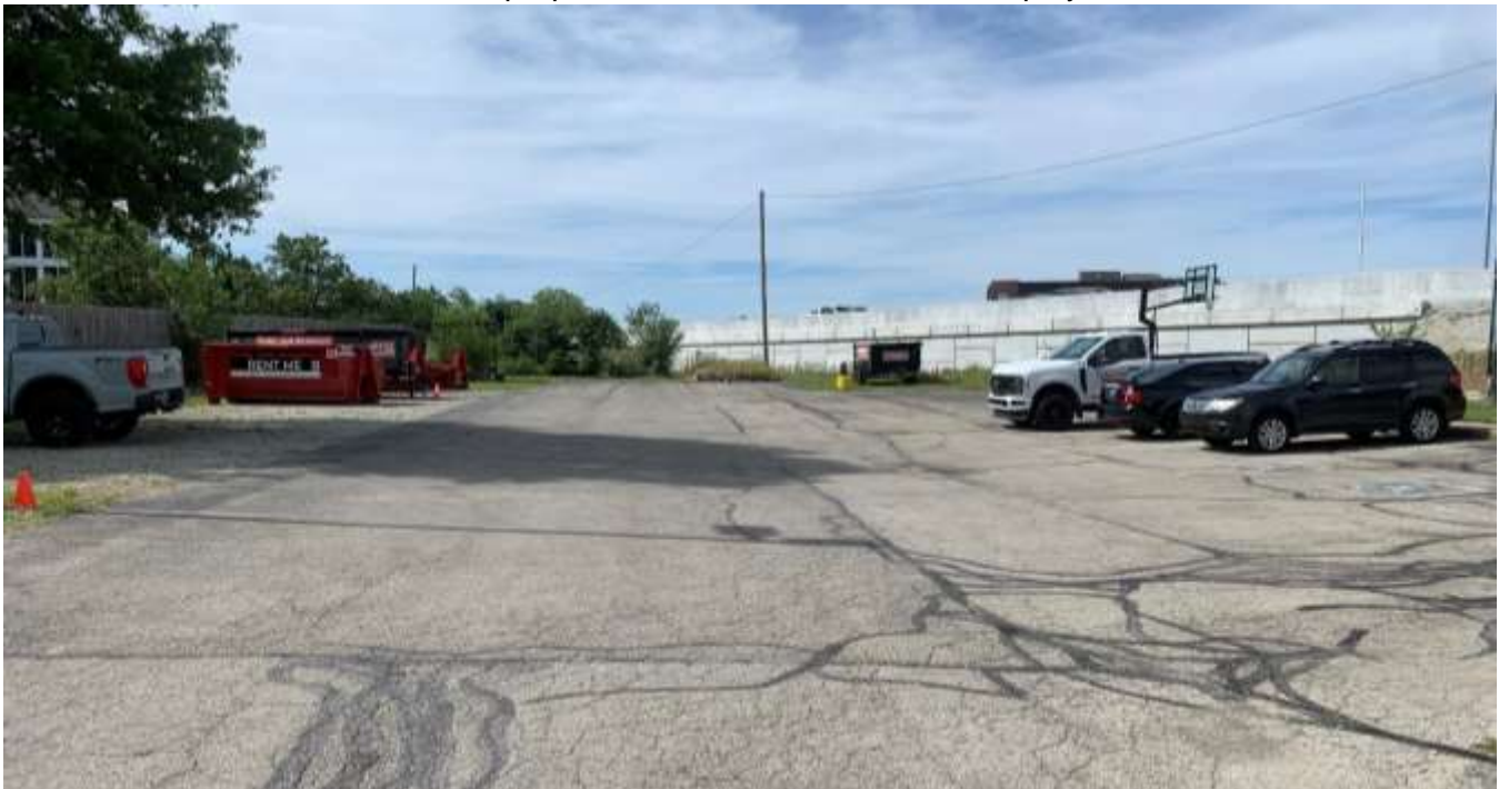
Photo of the remainder of the parking lot looking south.
