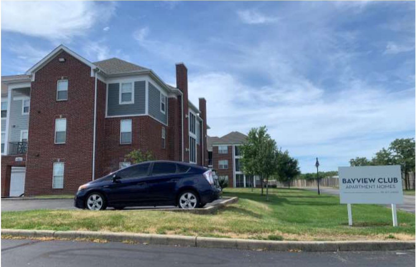
Photo of the apartment complex east of the site.
