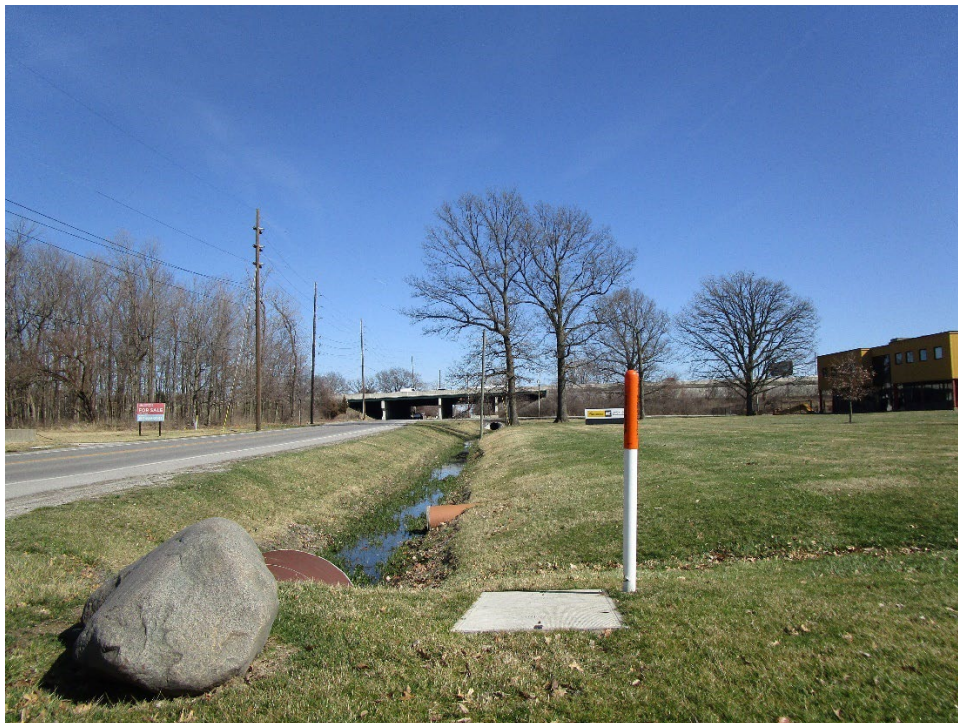
View looking east along East 30th Street
