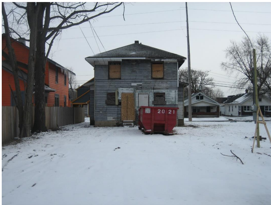
Photo 2- Subject property rear of lot, looking east.
