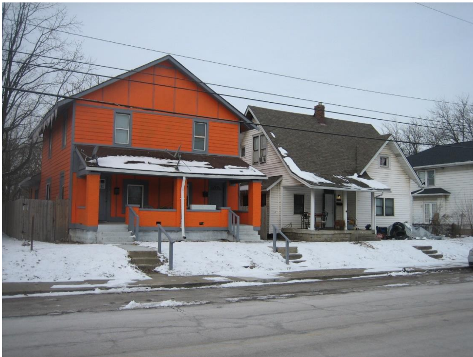
Photo 4- Adjacent properties to the north, looking northwest.
