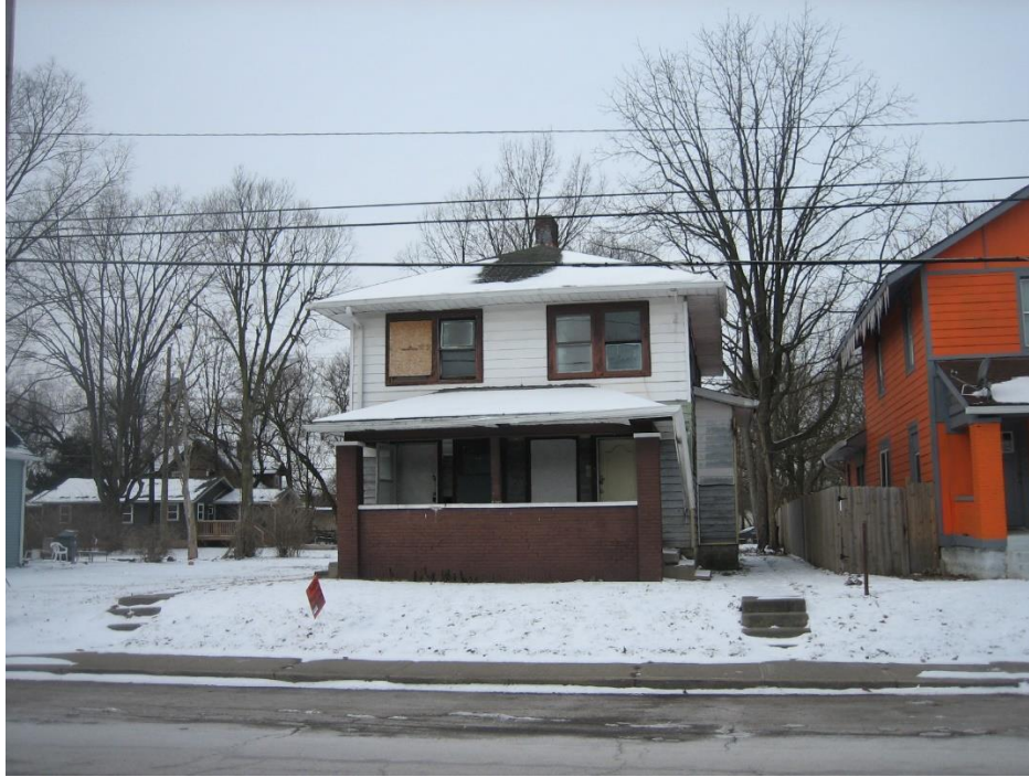
Photo 1- Subject property looking west.
