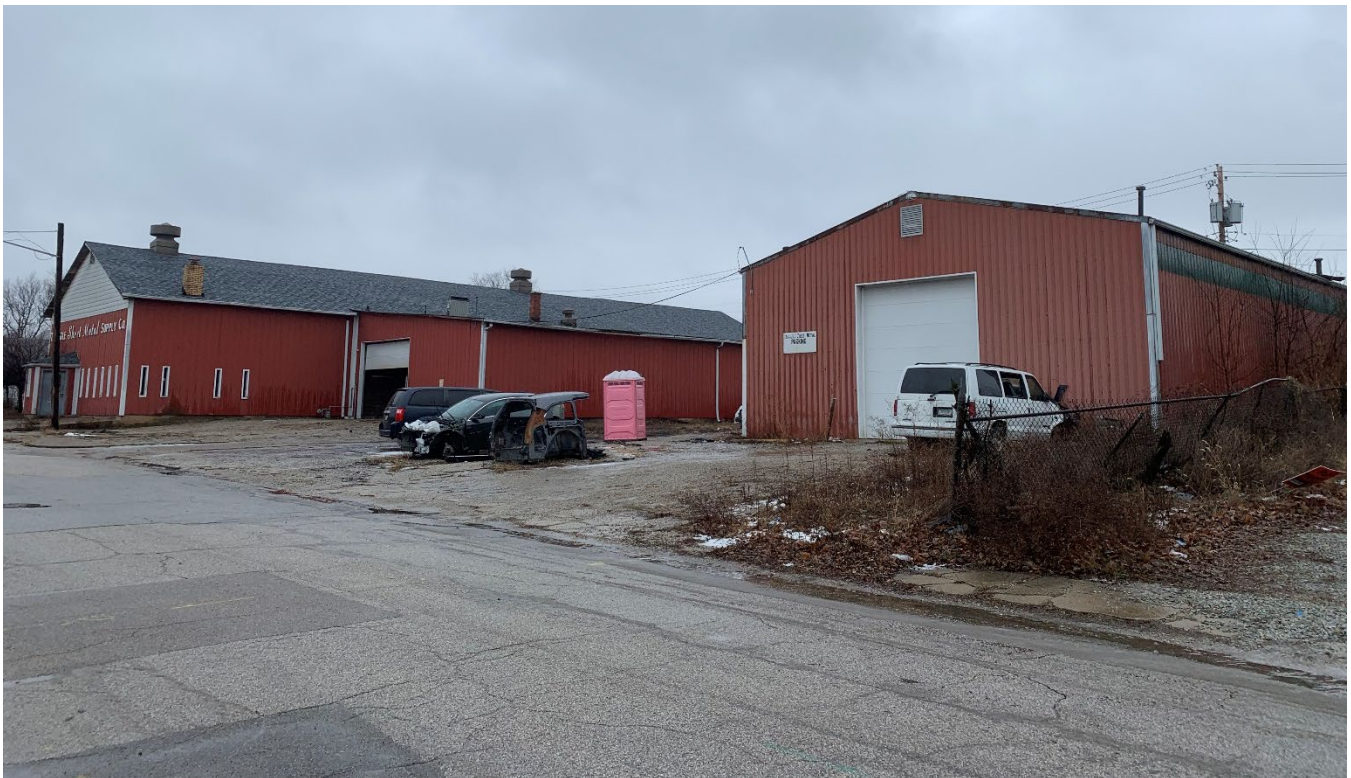
Industrial use to the north of the subject site
