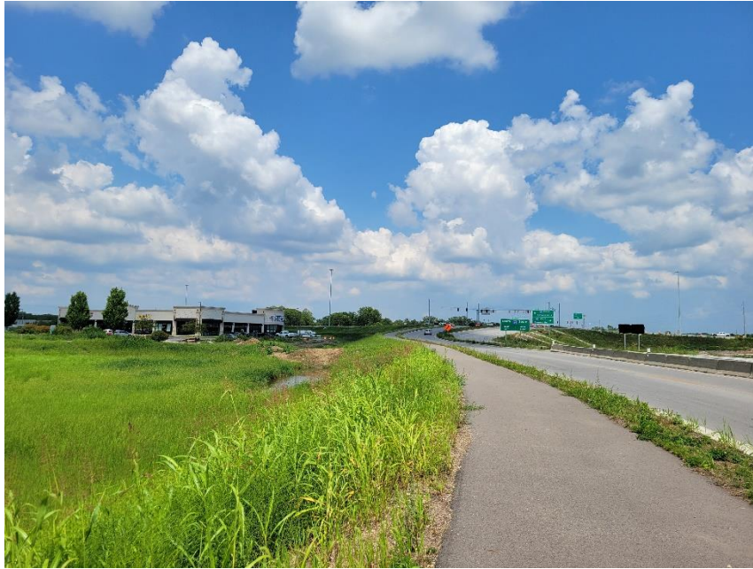
Photo 9: Recently Constructed Walking Path on Northern Side of Southport
