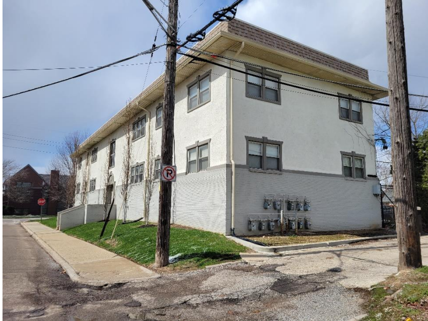
Photo 9: Adjacent Building to West
