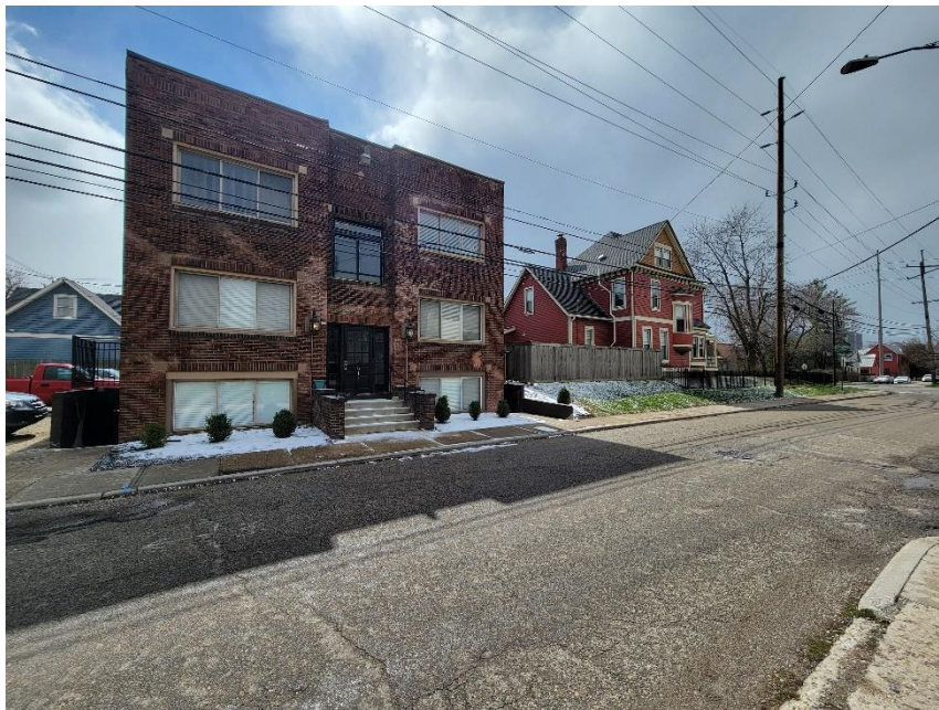
Photo 8: Adjacent Property to Southwest
