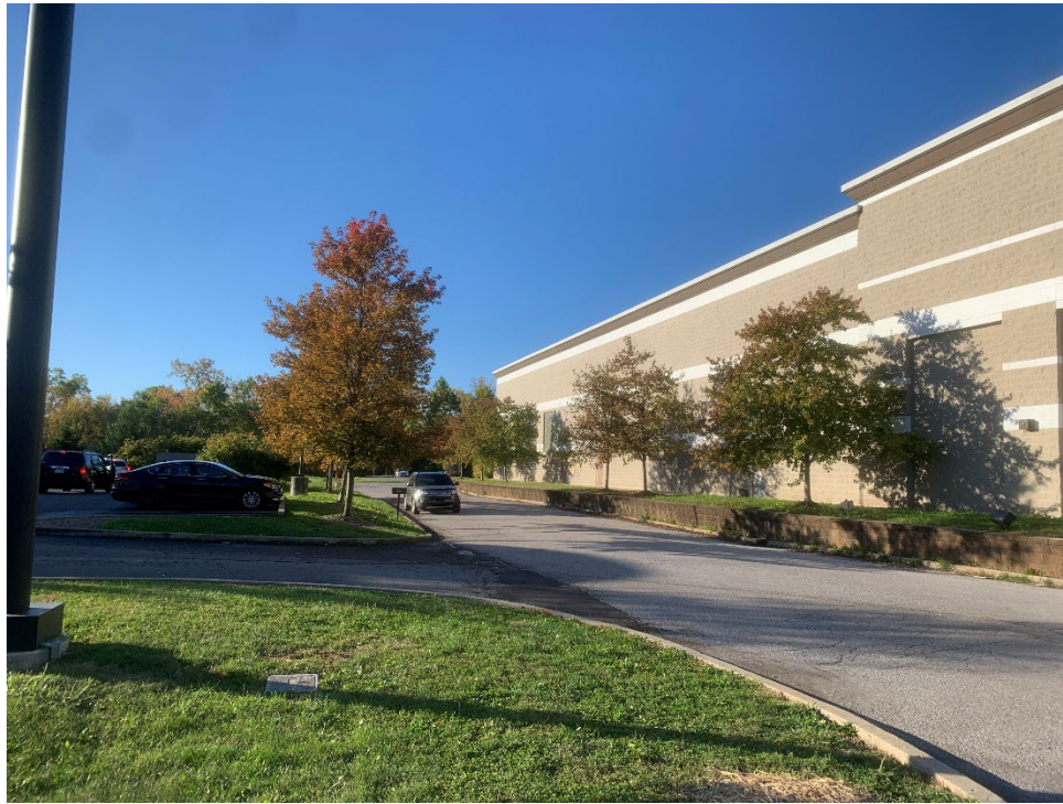
View looking south along western access drive
