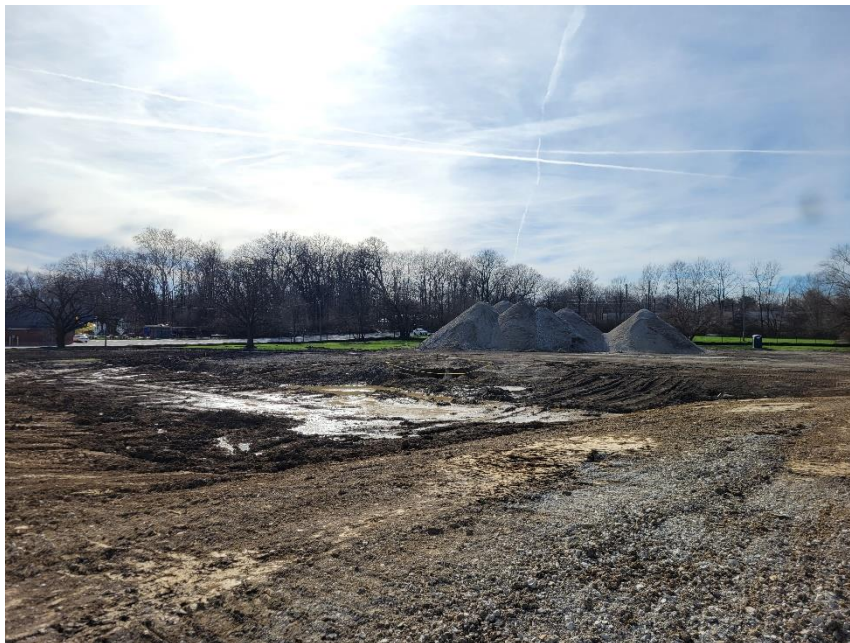
Photo 4: Site of Demolished Structure Viewed from Northeast
