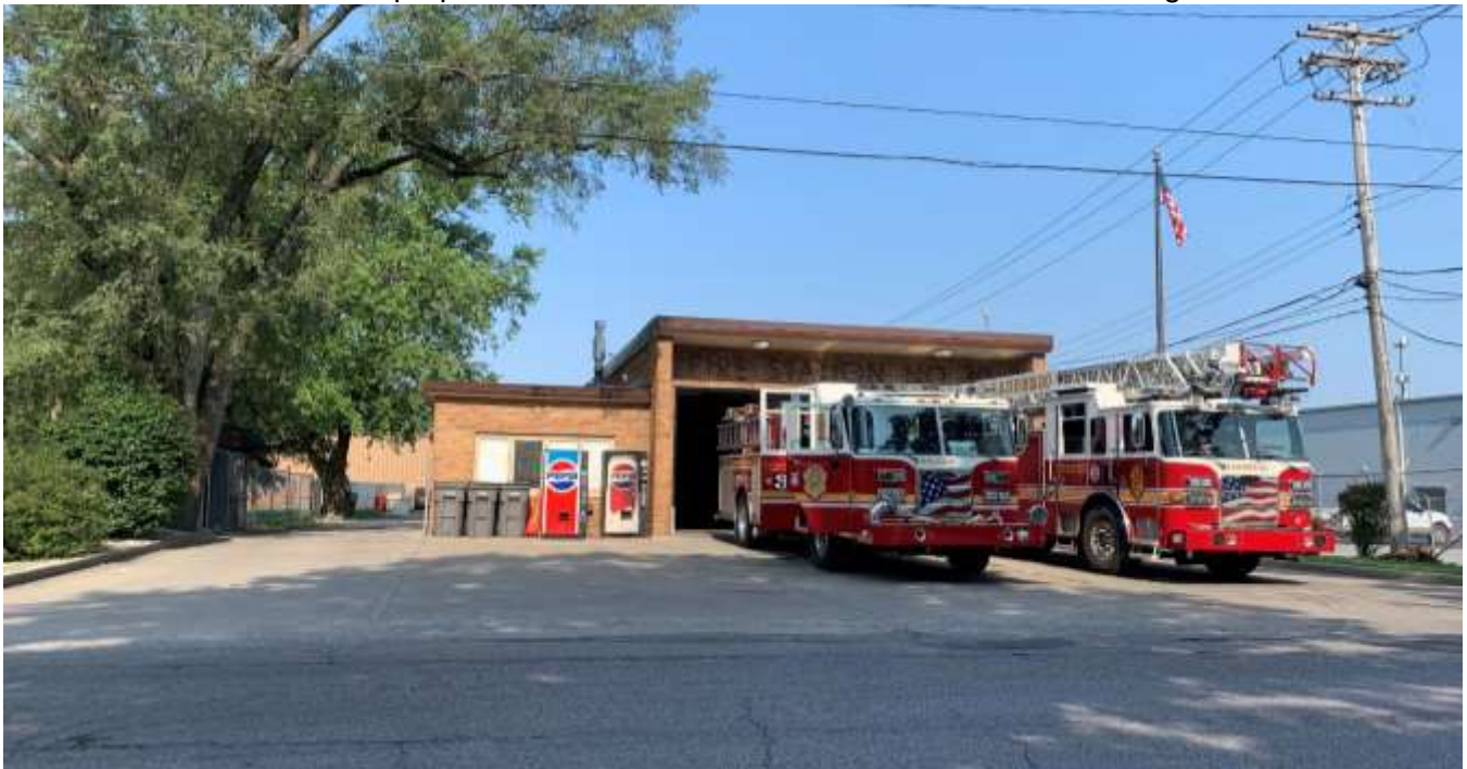
Photo of the existing fire station looking west.
