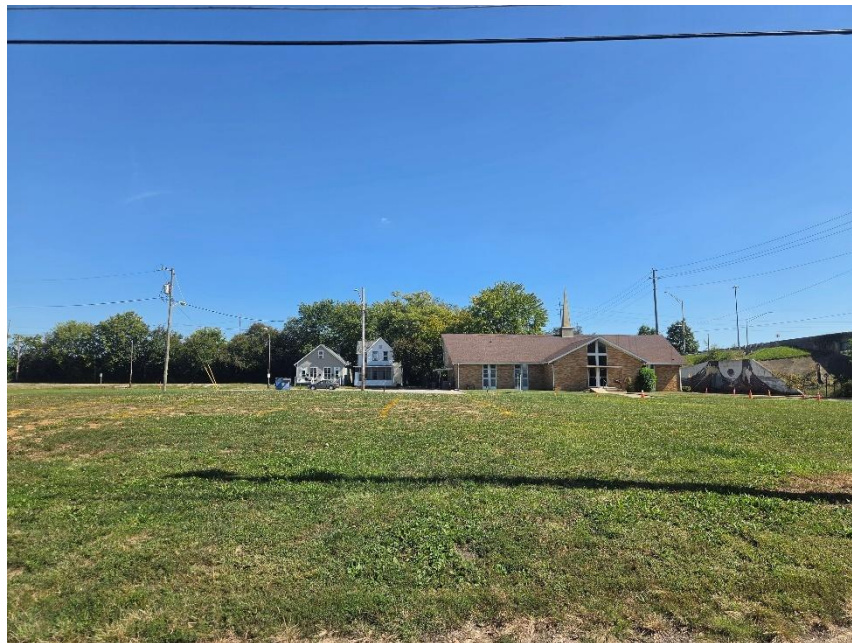
Photo 8: Adjacent Property to East
