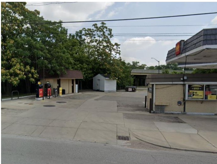
Photo 4: Subject Site from West (taken August 2023)
