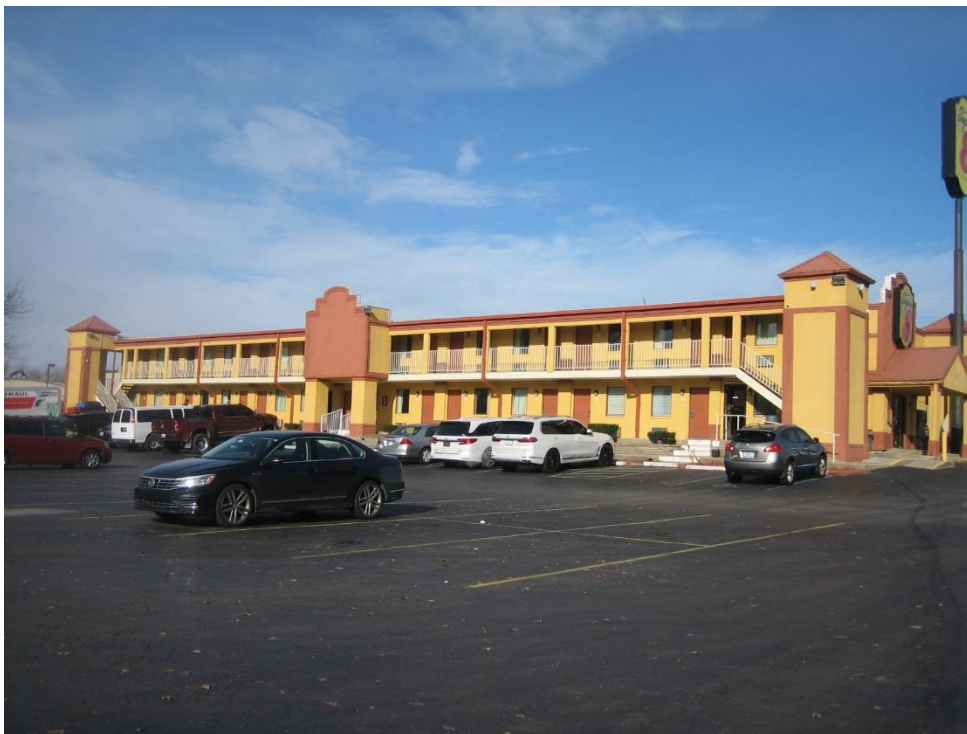
Subject site, south façade, looking north.
