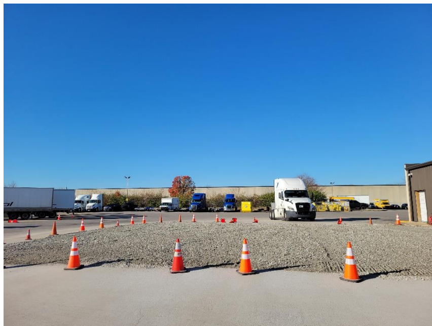
Photo 2: Previous Canopy Location viewed from East
