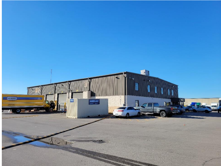
Photo 5: Primary Building Viewed from Northeast
