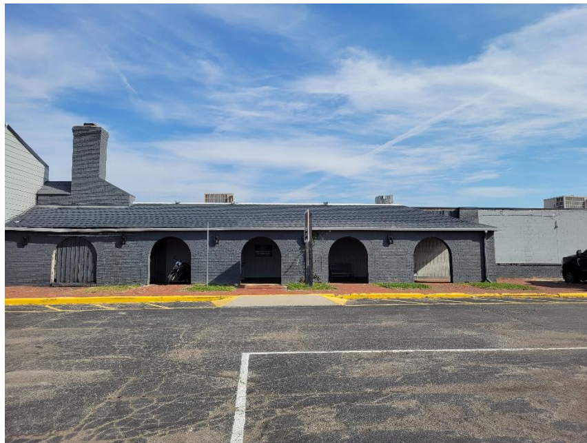
Photo 2: Subject Site from West (southern portion)
