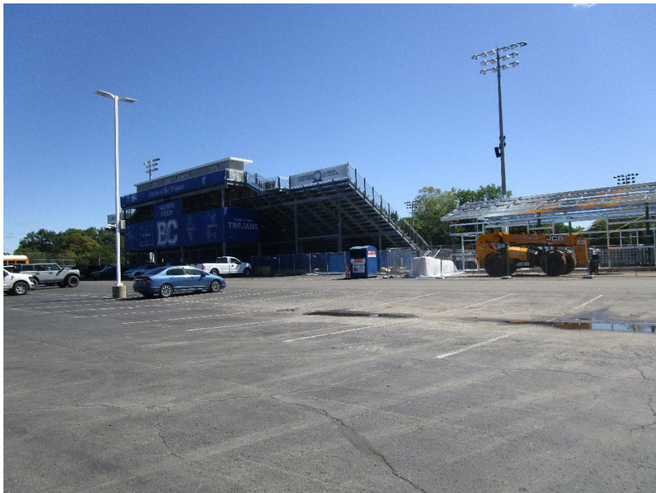
View of school campus looking northeast from East Crittenden Avenue
