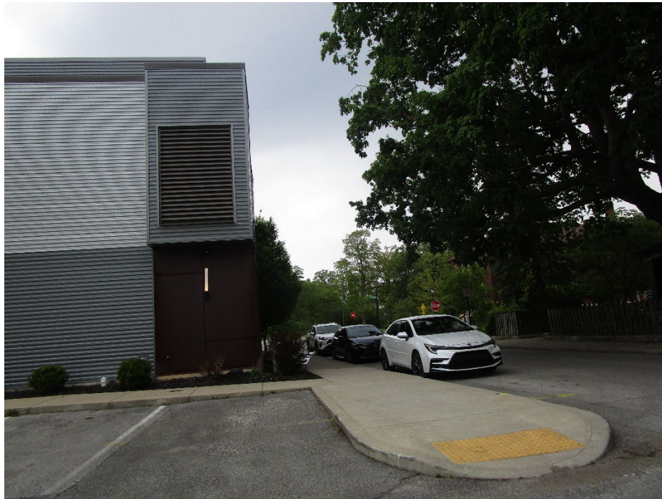
View of site looking north along Windsor Street
