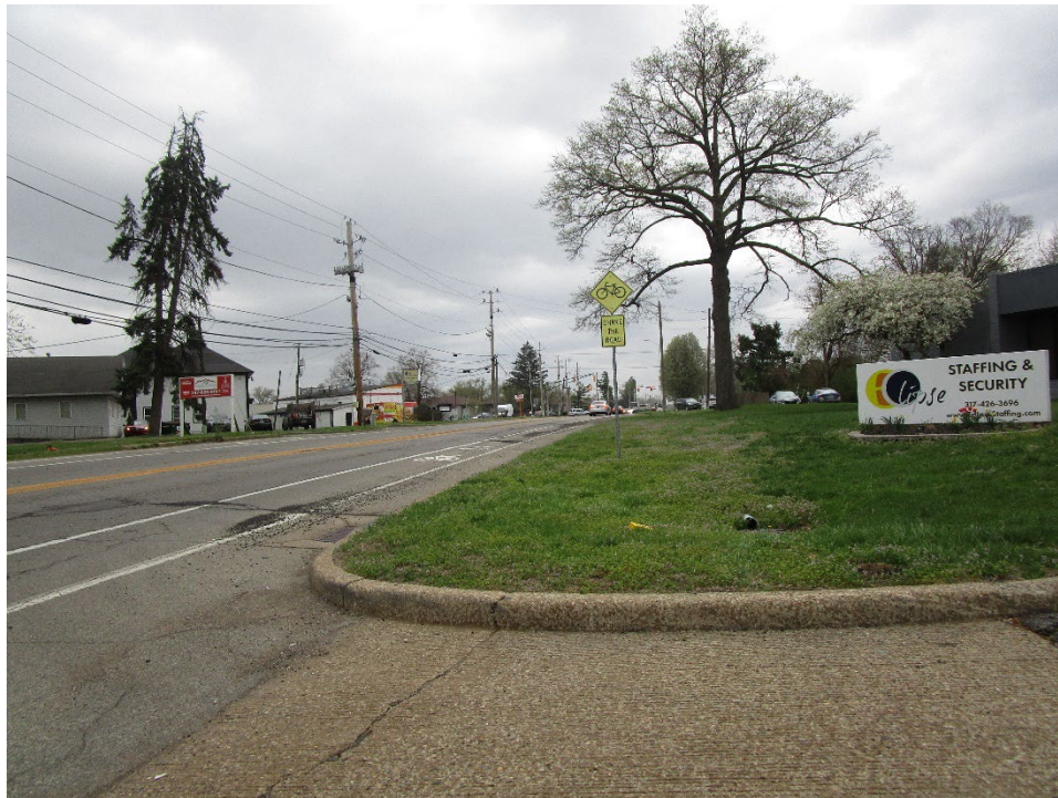
View looking north along Allisonville Road
