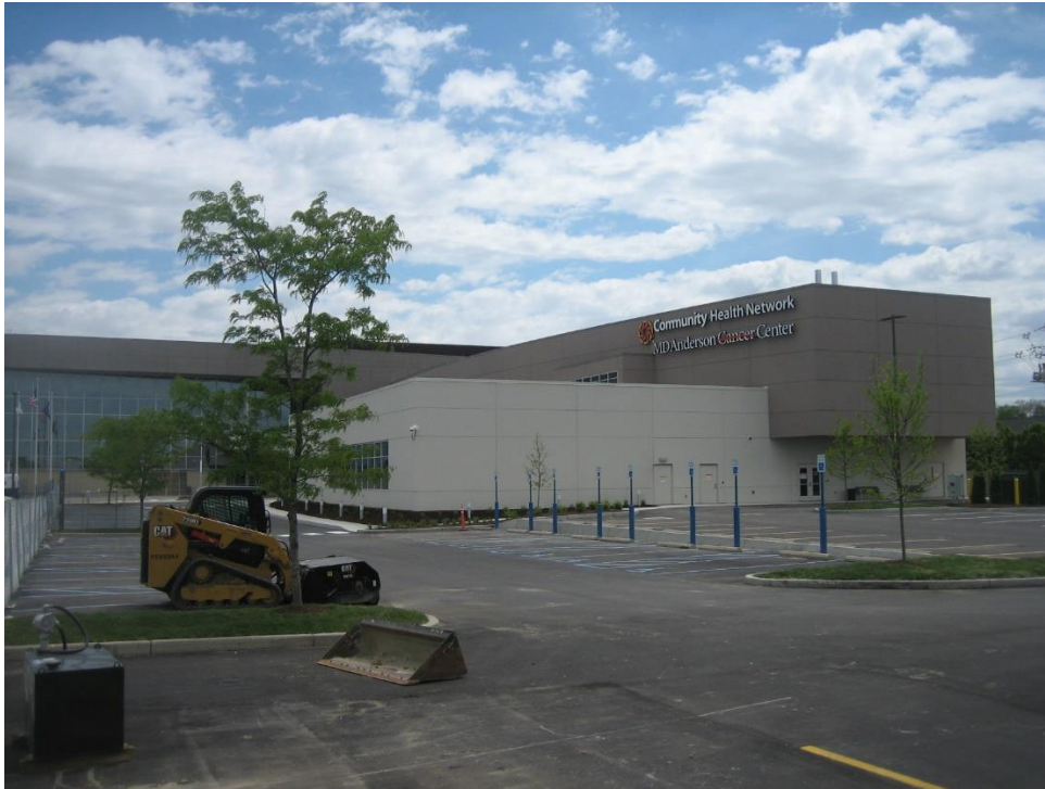
Photo of subject site, east façade, looking southeast.
