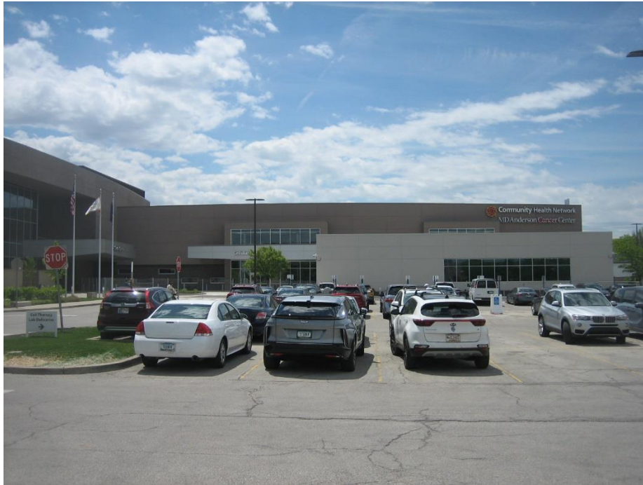
Photo of subject site, looking south at proposed sign location on north façade.
