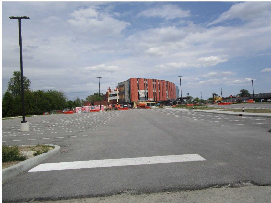
View of site looking northeast
