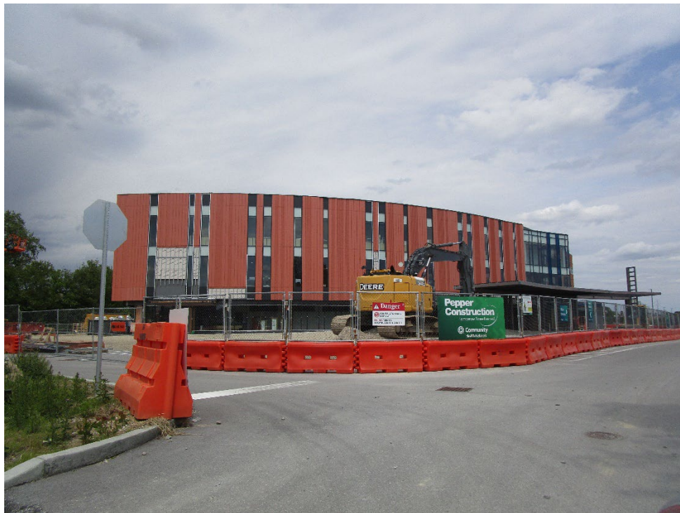
View of site looking northeast
