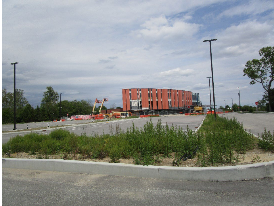
View of site looking east
