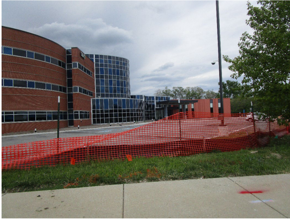
View of site looking east
