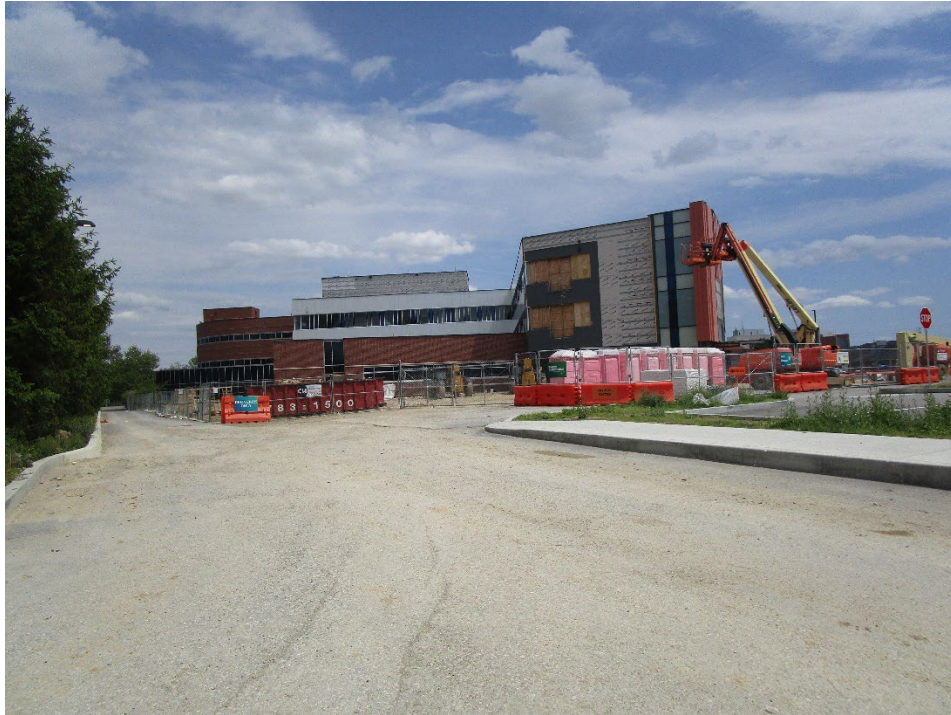
View of site looking east
