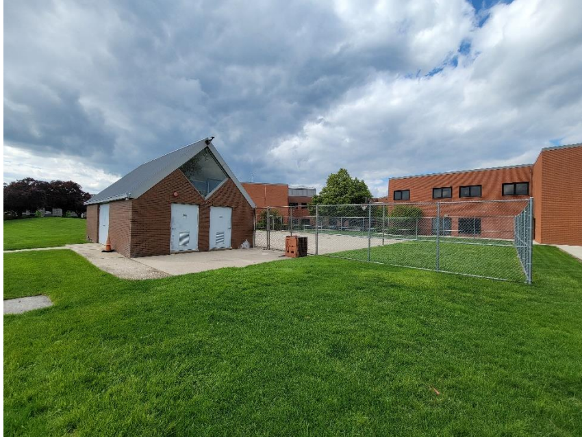
Photo 3: Subject Site Viewed from East
