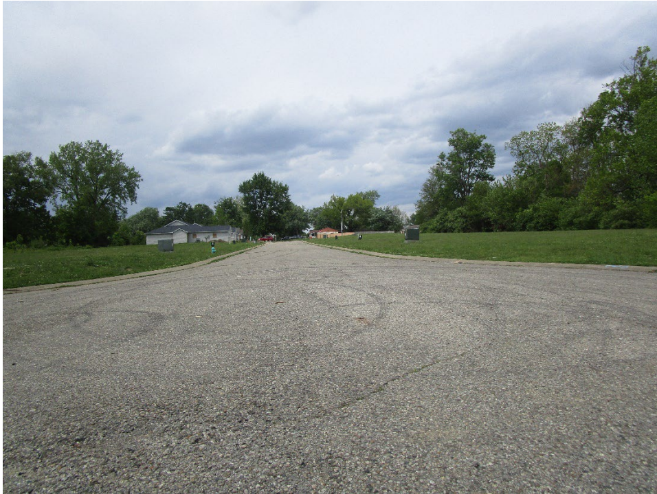
View looking north along Walker Place
