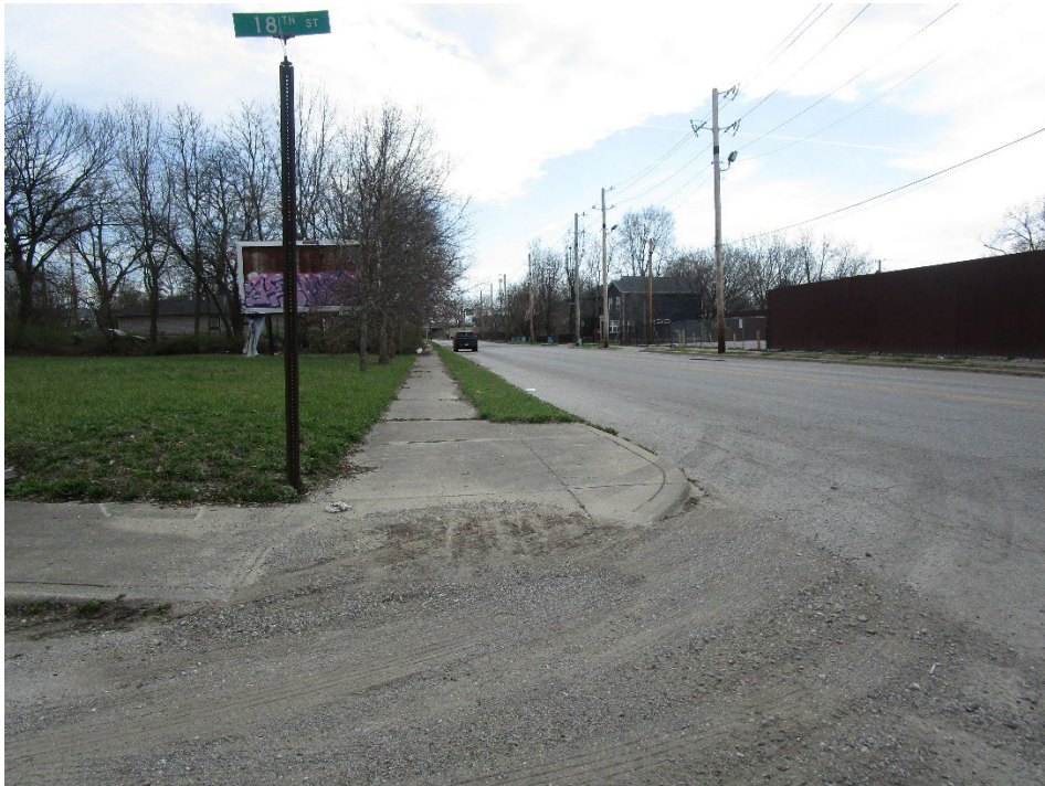
View looking south along Roosevelt Avenue
