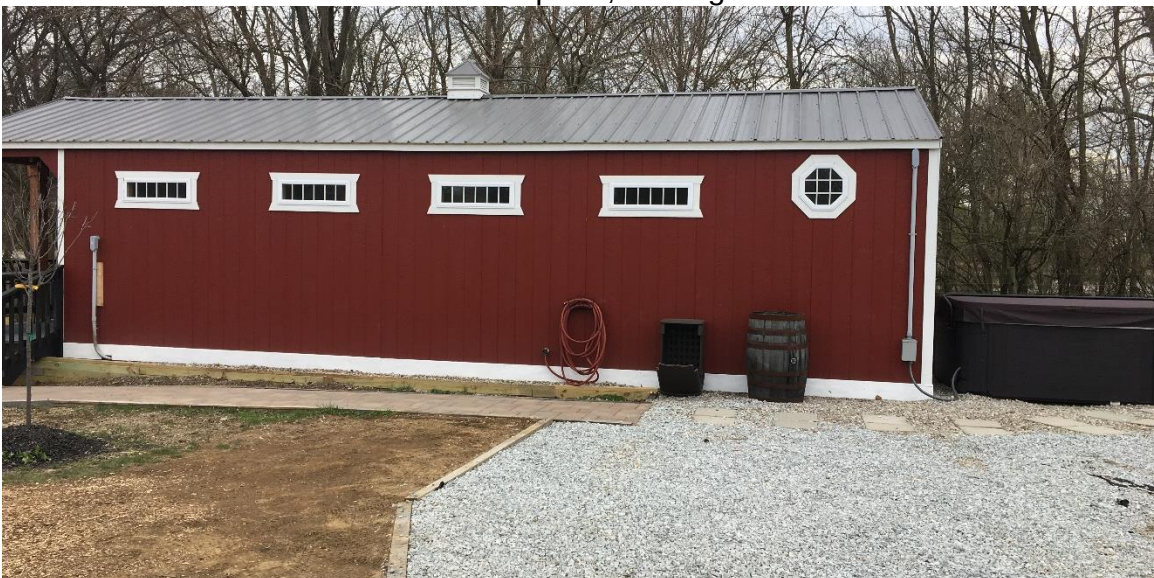
Secondary dwelling cabin, looking south
