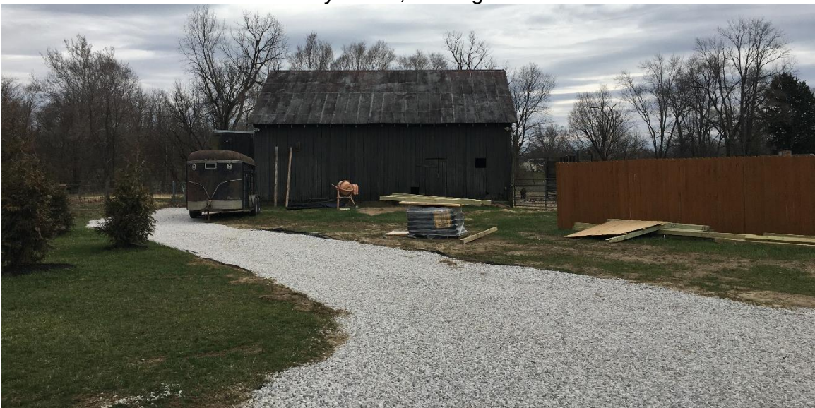
Existing barn, looking south
