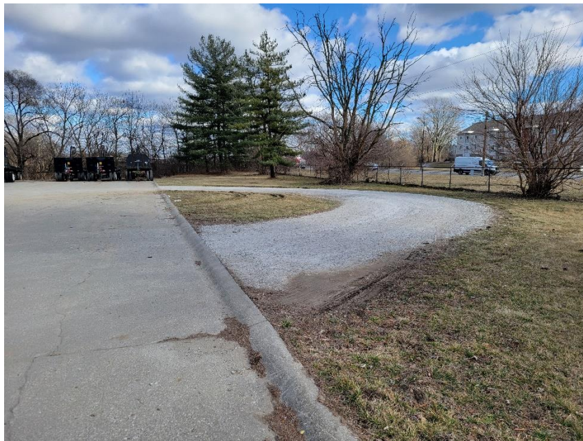
Photo 2: Horseshoe Gravel Area For Truck Maneuvering (Installed 2021)
