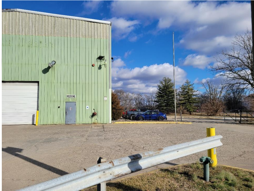
Photo 5: Truck Entrance Area & Partial Western Elevation
