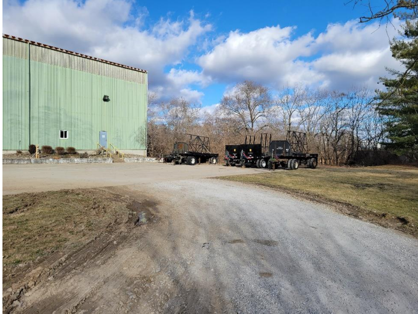
Photo 3: Partial Southern Elevation & Loading/Storage Area
