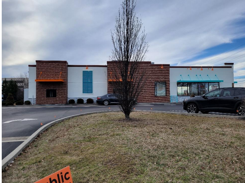
Photo 1: Eastern Elevation (Front Yard)
