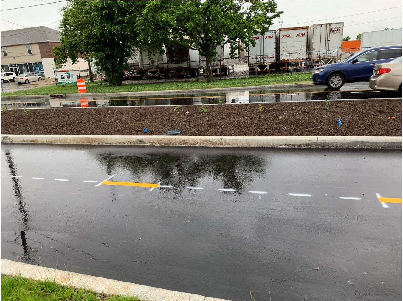
View of bike lane, landscape buffer zone and the two travel lanes of Michigan Street
