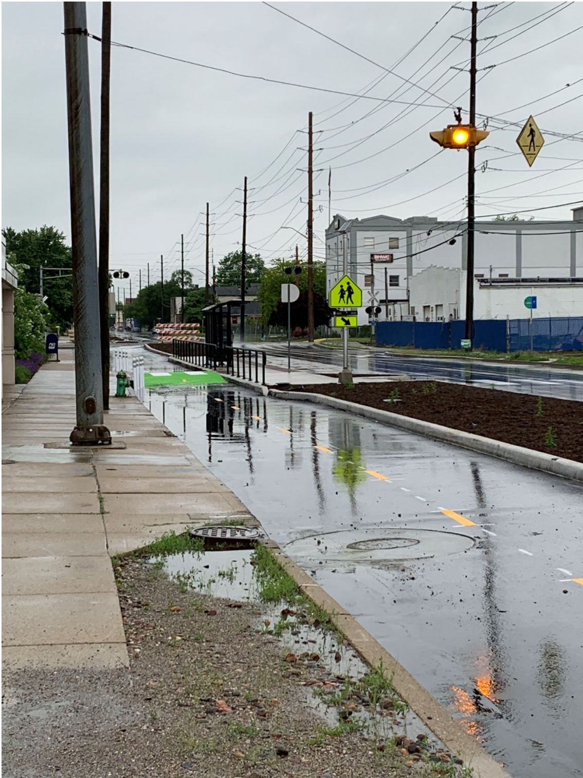
Close-up view of bus stop, bike lane, landscape buffer zone and the two travel lanes of Michigan Street, looking west
