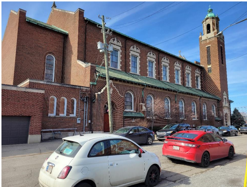
Photo 10: Adjacent Property to South
