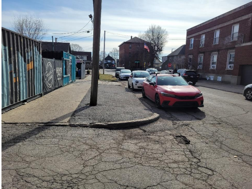
Photo 5: Bicycle Parking Area & St. Patrick Right-Of-Way
