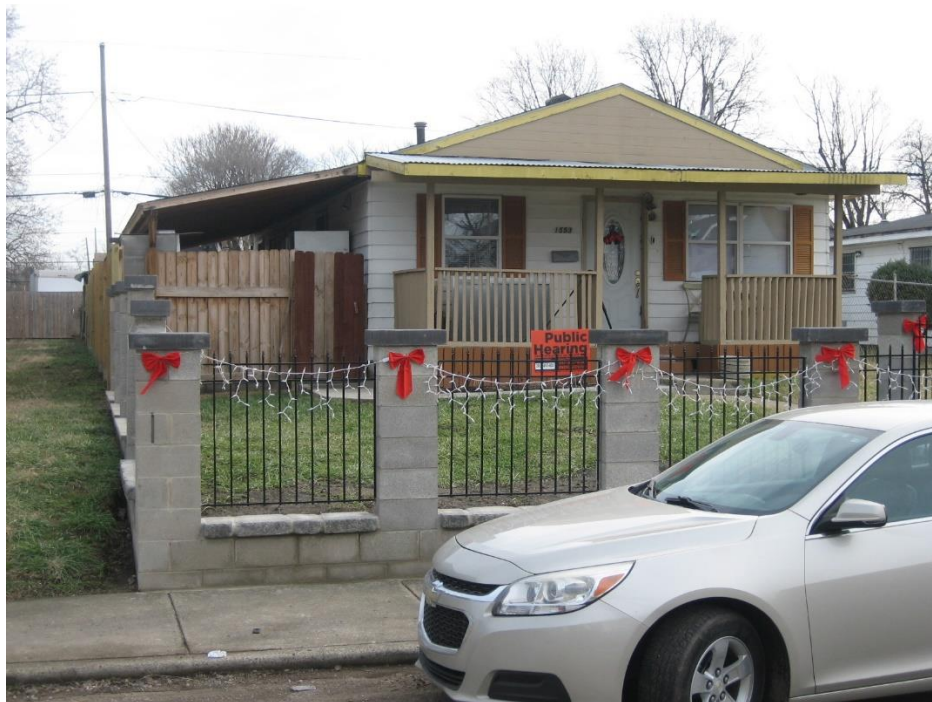
Photo 2- Subject property attached covered porch with zero-foot north side yard setback, looking east.
