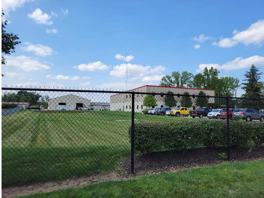
Photo 7: Adjacent Property to North/Northeast (viewed from Massachusetts)
