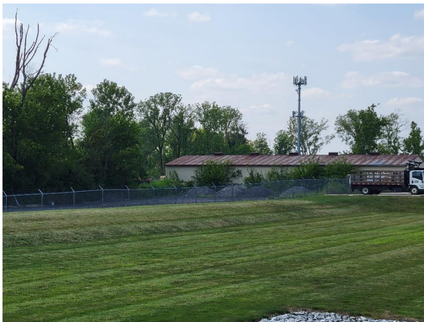
Photo 4: Rear of Subject Site Viewed from East
