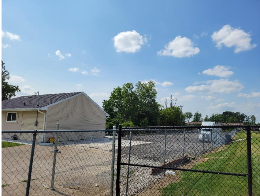
Photo 5: Fence at Subject Site (D-3) and Adjacent Property (I-3)
