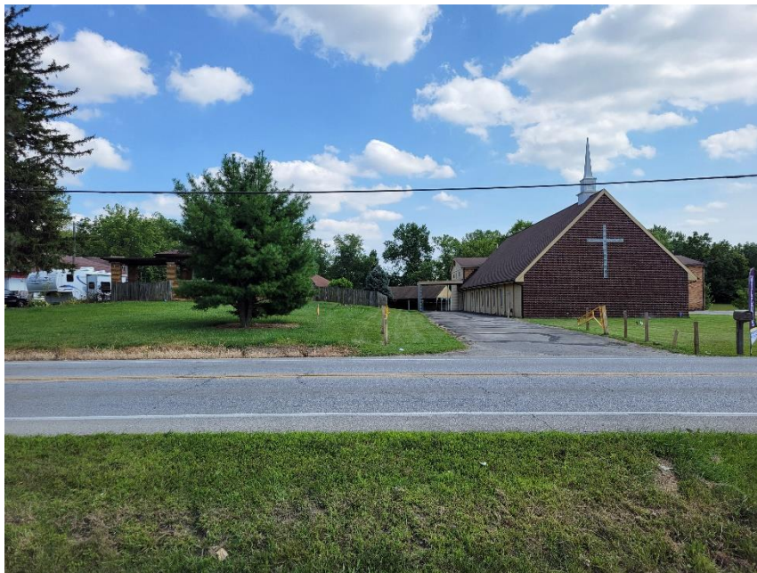
Photo 8: Adjacent Property to Southeast
