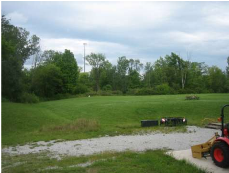
Subject property septic field and drainage swale to the rear of dwelling, looking east.
