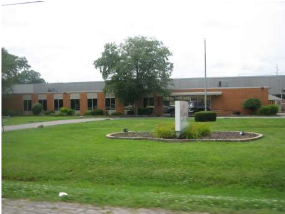
Adjacent industrial property to the south, looking west.
