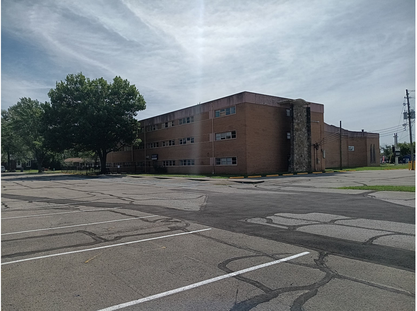
Exhibit 6: North left-side of the church building, facing southeast.
