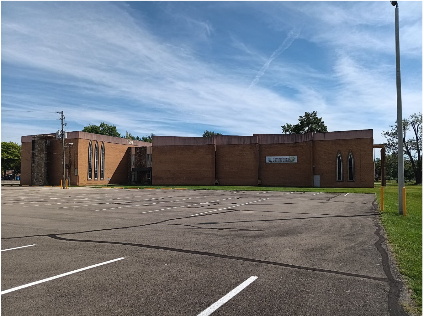
Exhibit 7: West side of the church building, facing east.
