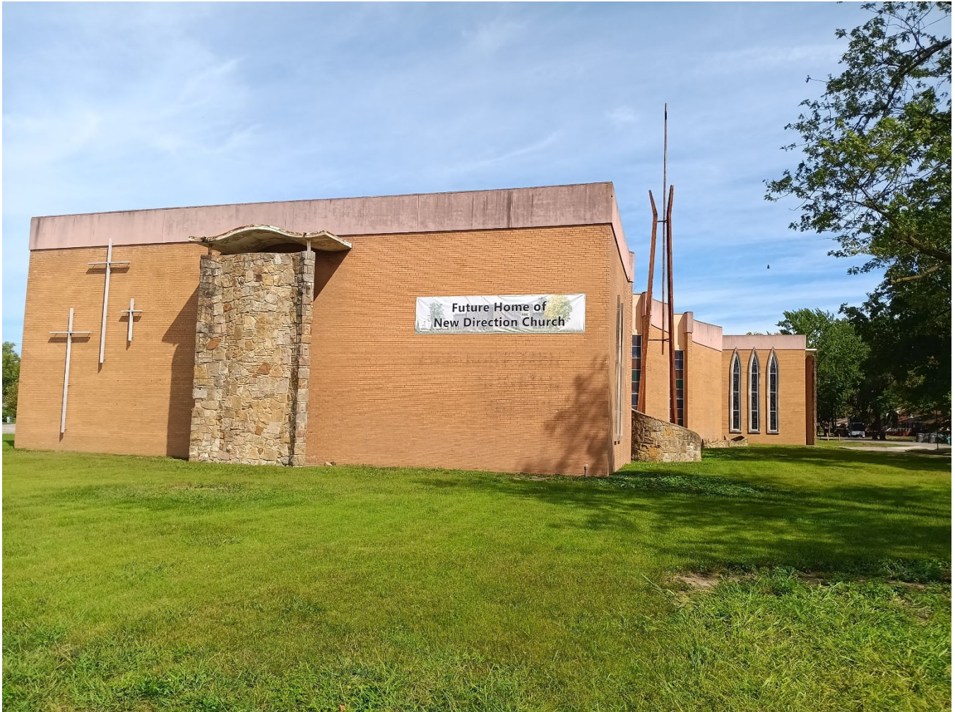
Exhibit 8: South and east side of the church building, facing north.
