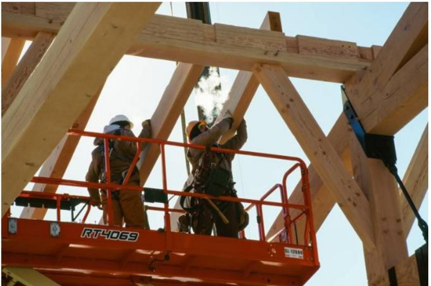
The Crew Worked Tirelessly Through Bitter Cold For This Raising
