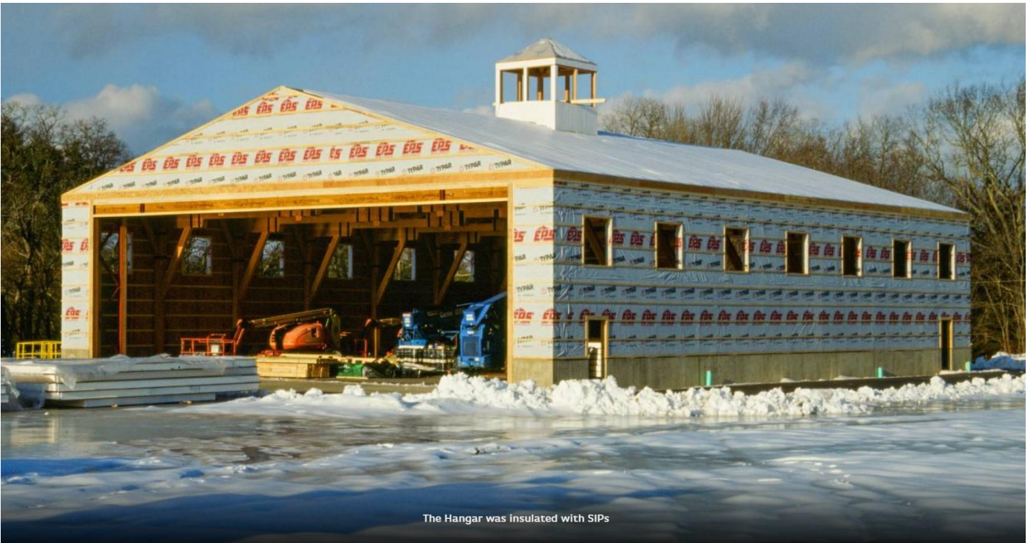
The finished frame with roof decking
