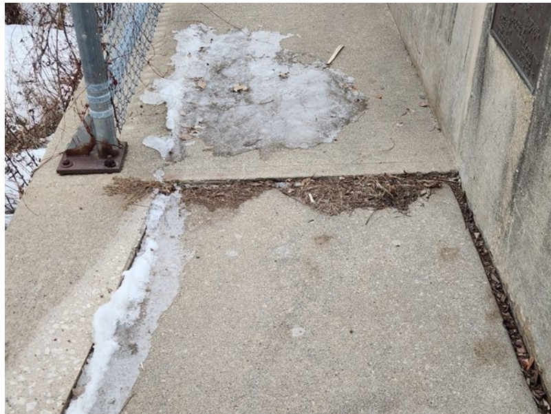
File Description Sidewalk approaches settling
