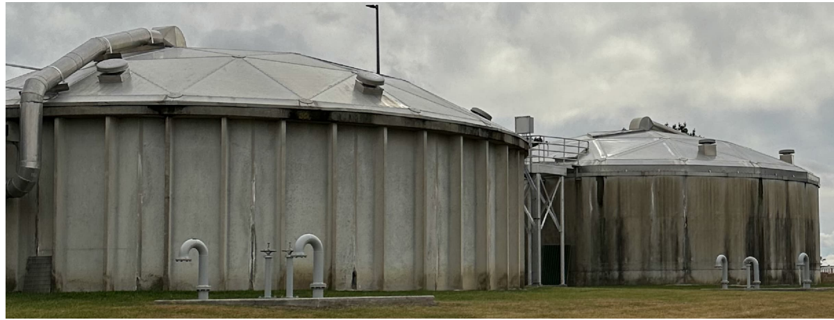
Existing Trickling Filters
