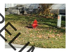
Fire Hydrants located throughout the community will need to be reconditioned. This category is to recondition these hydrants. Not all components will need to be replaced but inspection and replacement of seals and other deteriorated components as needed.
