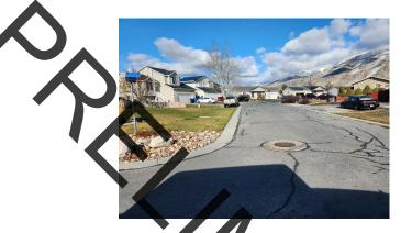
The streets are in fair condition for the age, however, there are signs of cracks and deterioration. Regular sealing may prolong the bre of this component. Streets replacement includes removal and replacement of the exiting asphalt. This replacement does not include extensive work to the base material. Some repair or replacement of the curbs may be needed but full replacement of the curbs is not included in this estimate.
