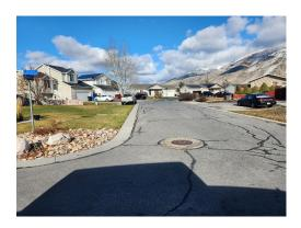
The streets are in fair condition for the age, however, there are signs of cracks and deterioration. Regular sealing may prolong the life of this component. There are various methods and treatments to protect and preserve the asphalt. Consult asphalt professionals to determine what treatment is going to be the best for your asphalt.
