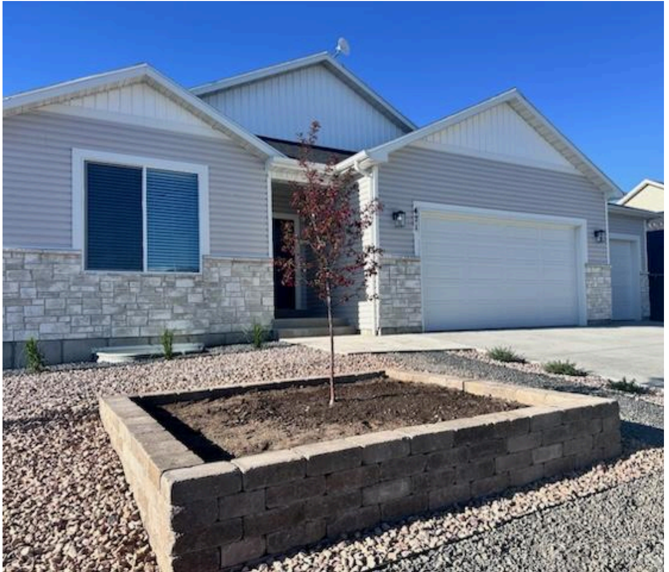
Image D: Front View of House
